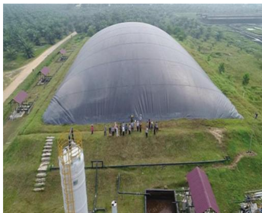
Figure 13.1 The government continues to encourage the development of renewable energy to be utilized massively by developing the potential for palm oil effluent or POME as a raw material for biogas which can be used as fuel for power plants.
