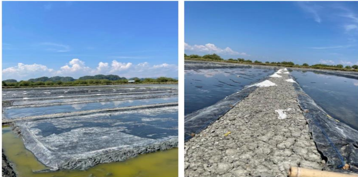
Figure 2.5 Salt ponds in Bulu Cindea Village, Bungoro sub-district, Pangkep Regency: (a) Use of geomembrane technology; (b) Salt production using geomembrane technology
